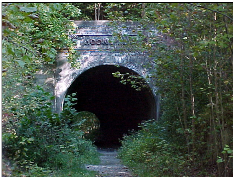
Figure 3. Picture of Moonville Tunnel
