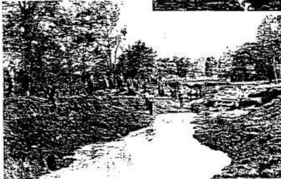
Straightening of Pequest River in New Jersey by CCC workers stopped its yearly floods. Location of new channel is seen at right. Note temporary dam at left to provide volume of water for scouring blasted channel.
